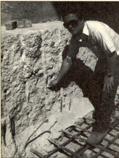
After completing its expansion, the S-Mite turns into a powder which can be brushed away. The exposed mat rebar is visible at the bottom of the photo.
