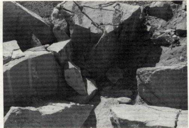
Figure 4 - Fractured boulders 24 hours after loading with S-Mite.
